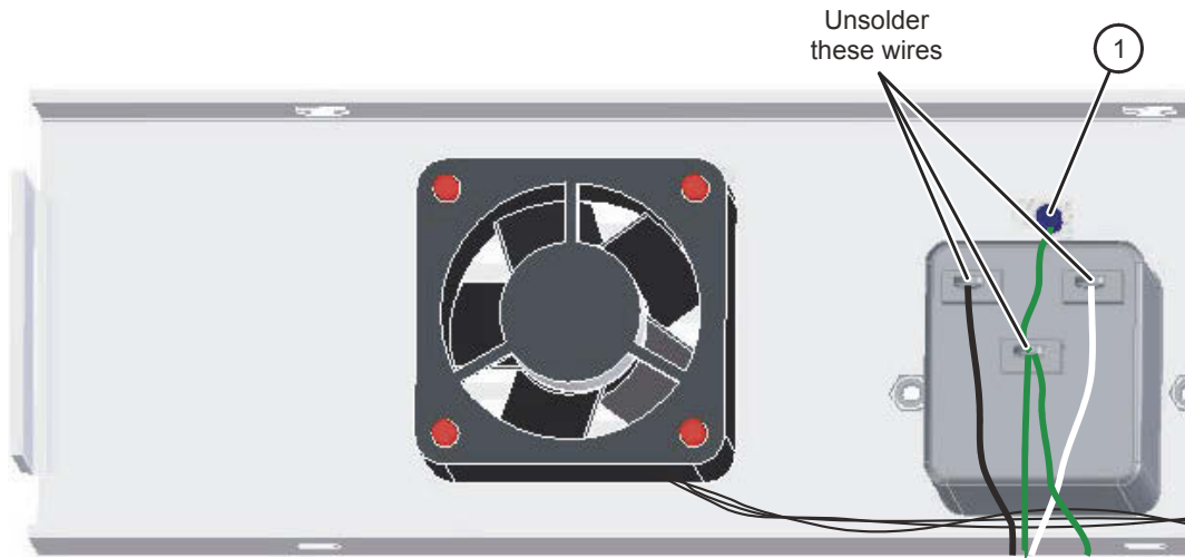
Figure 7-14 AC Line Module Removal
