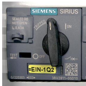
Transformer circuit breaker for Measurement & Control Unit (MCU) (=EIN-1Q2) (illustration similar)
