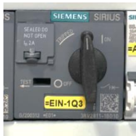
Transformer circuit breaker for 24 V power supply (=EIN-1Q3) (illustration similar)
