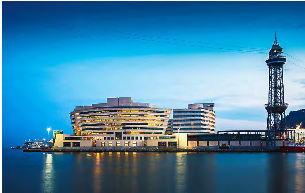
Keysight facility in Barcelona, Spain
