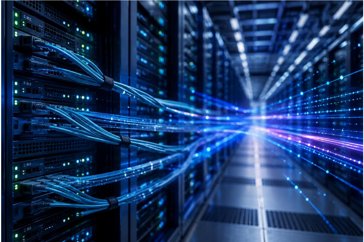
Figure 1. AI scale-up architectures are driving critical bandwidth, power, latency, and reliability challenges across hyperscaler data center interconnects
