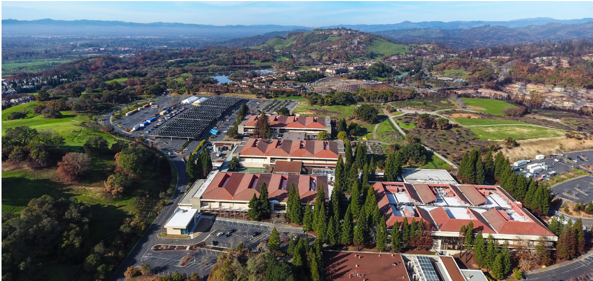
Keysight facility in Santa Rosa, California (corporate headquarters)
