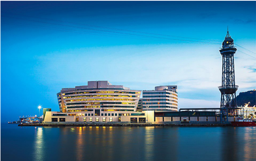
Keysight facility in Barcelona, Spain
