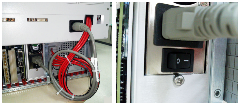
PXIe subsystem power switch (DUT interface view)
