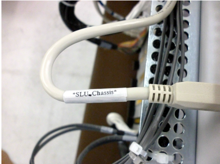
Figure 1-17 Interface cable label example (*SLU_Chassis*)
